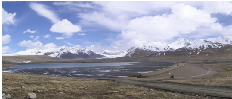
Figure 1. Kumtor tailings dam
